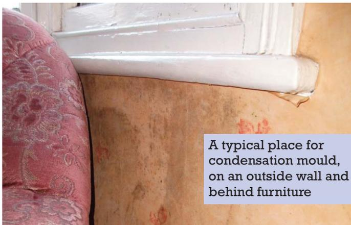
A typical place for condensation mould, on an outside wall and behind furniture
